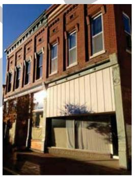
Various stages of facade restorations are needed along 4th Street. The building shown here is in good condition but needs the former storefront glass and casing replaced (photo taken 2013)
