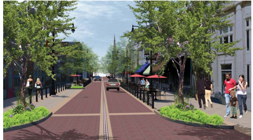
Center trench drains and bioswale planters collect the stormwater runoff and help to delineate the areas where flexing of the street can occur.
